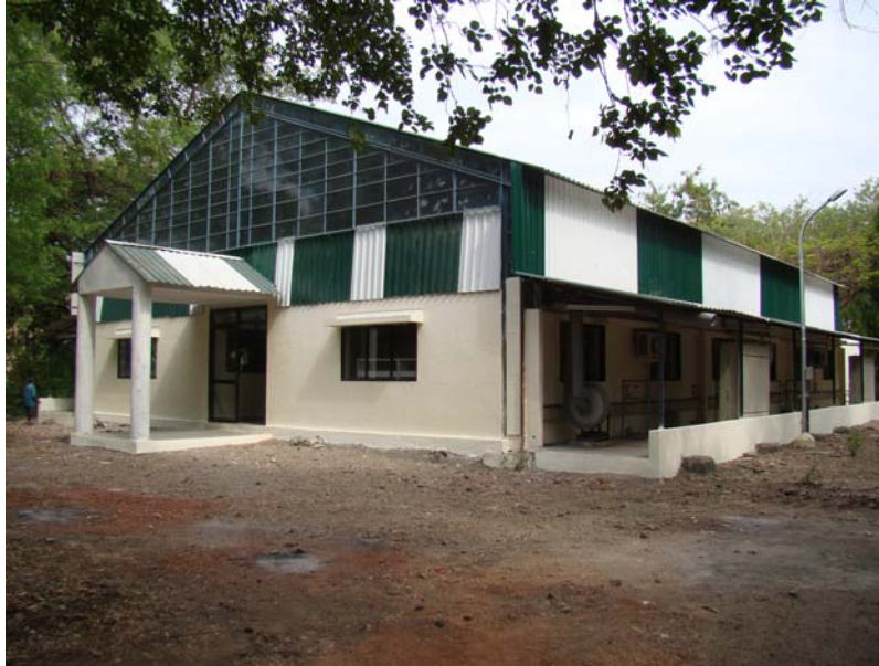
External View of Lab Block showing Service Corridors
