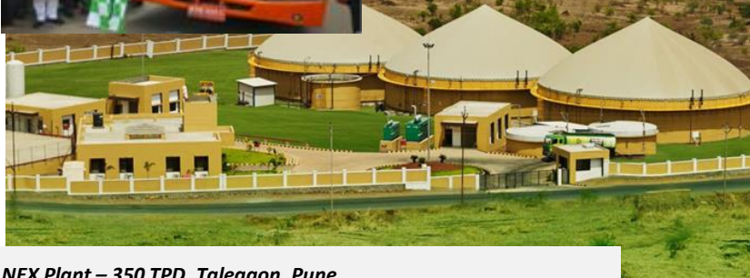
NEX Plant – 350 TPD, Talegaon, Pune
